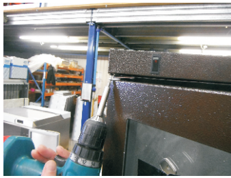
Remove screws holding the front of the lid in place
